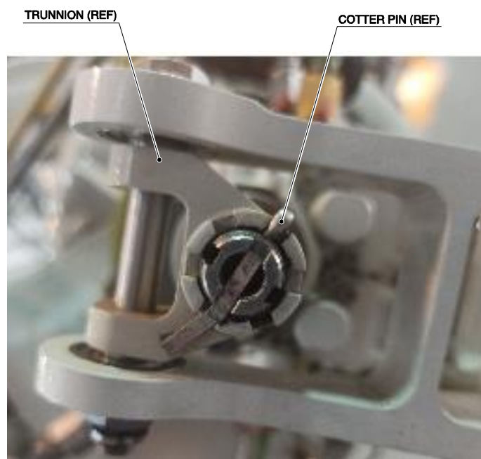
CORRECT COTTER PIN INSTALLATION WITH NO SIGN OF ROTATION VIEW B
