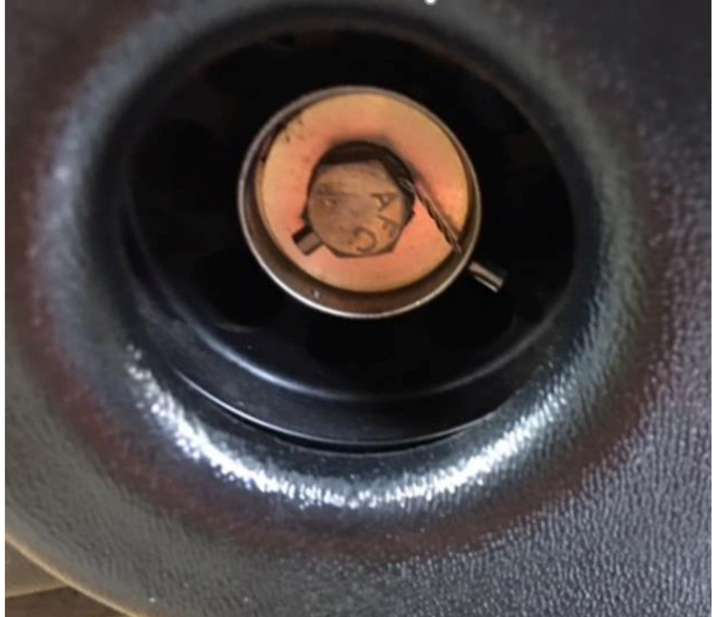
Figure 3: Drive Pulley Washer Installed
