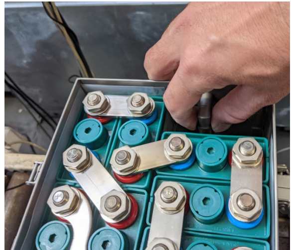
Figure 002 – Detailed view one-way valve (370) location and clearance for handling.
