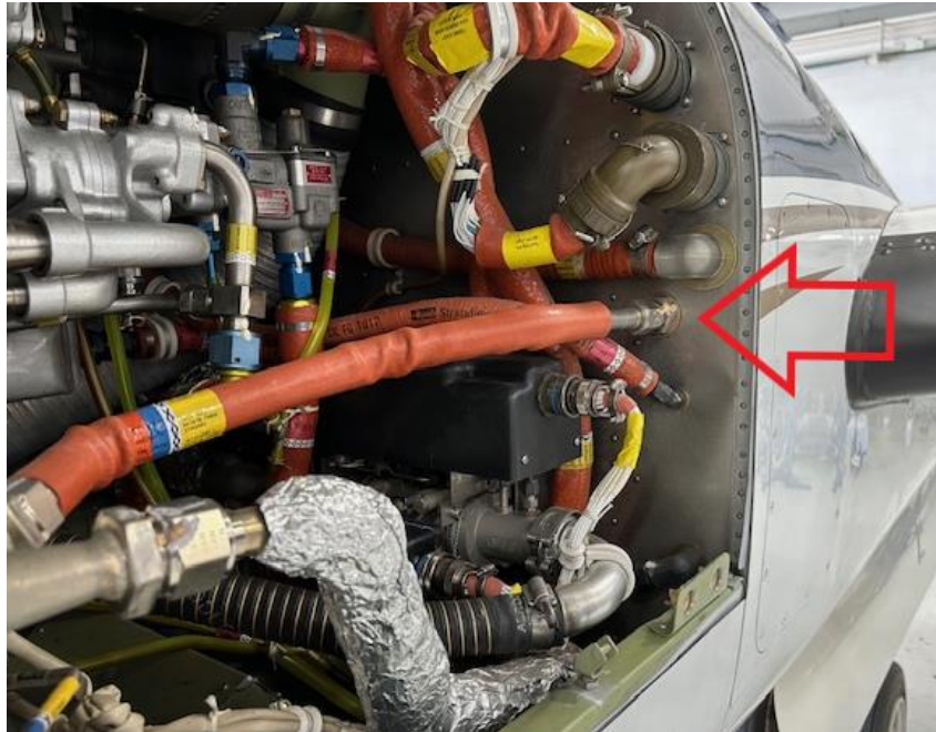
Line from “Y” from Engine Bleed Air Take-Off to Firewall Models B200/300/B300
