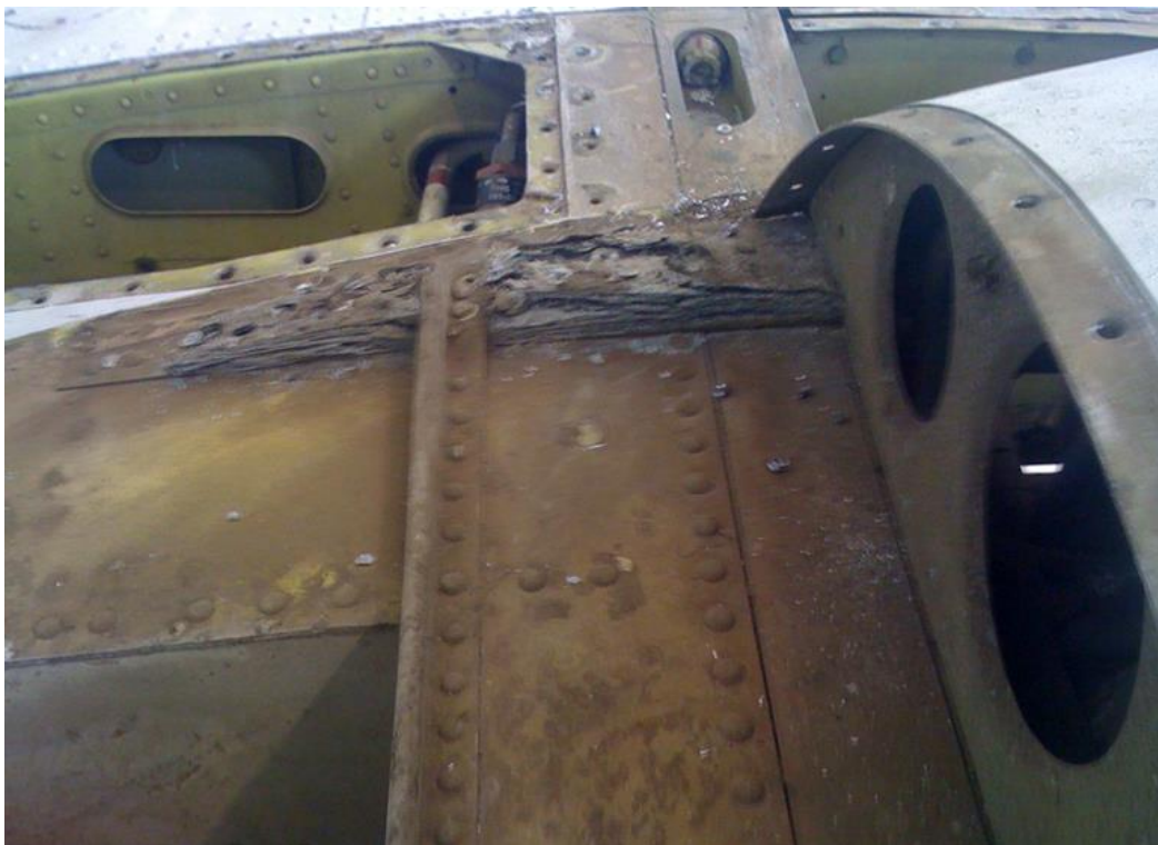
A Severely Corroded Example
