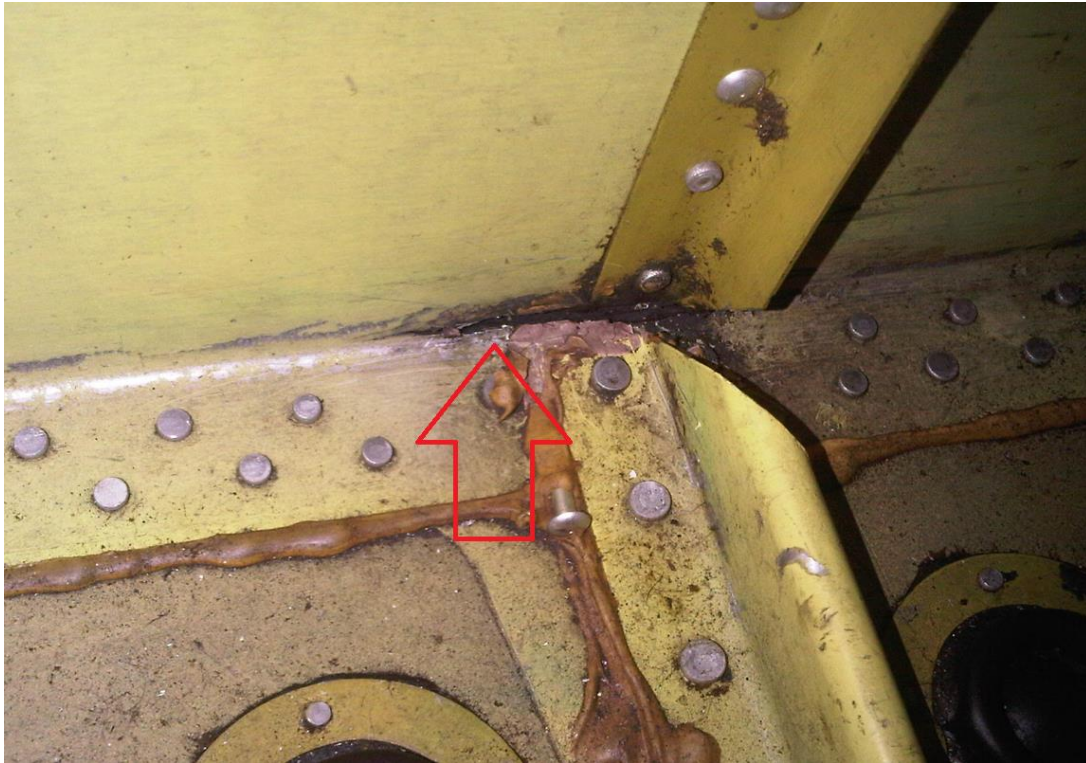
Main Spar Assembly Looking Forward At Aft Seal Plate
