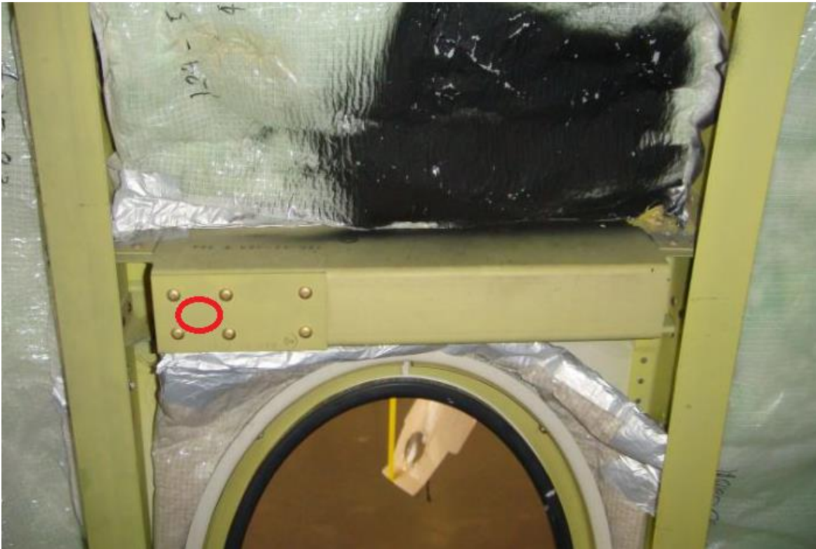
Closeup View of a Reinforcement Before Hole is Drilled
