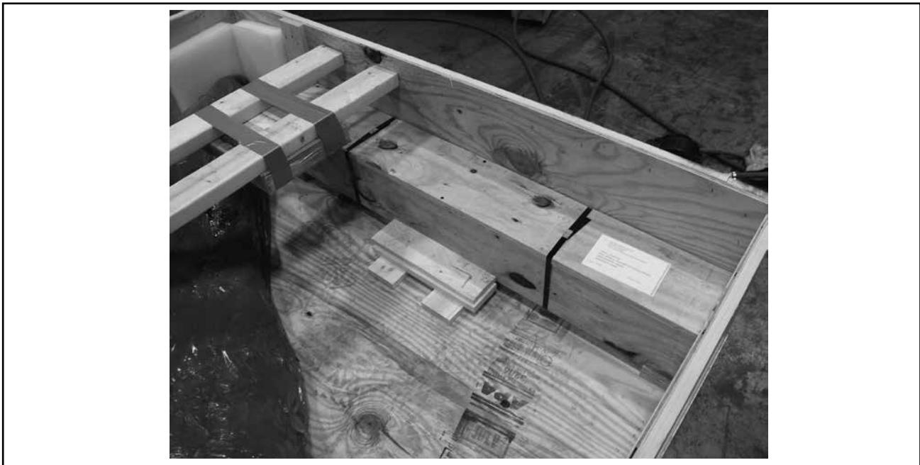
Securing the Box Containing the Beta Valve Assembly Figure 3-6
