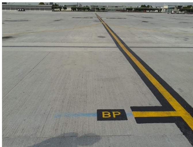
Figure 10-2. Aircraft Engine Start-up Position Line Marking
