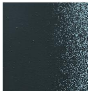
Not acceptable: P20 primer partly covered
