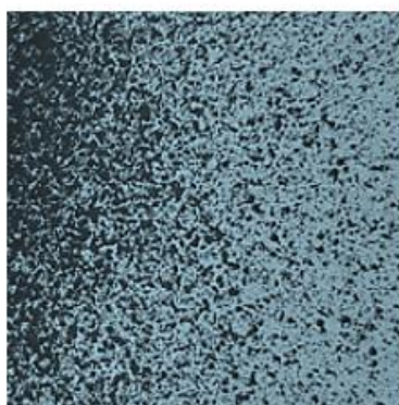
Acceptable: P20 primer exposed across the whole surface
