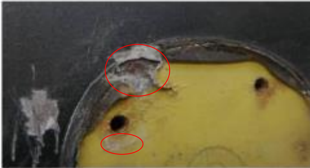
Example of corrosion and aluminium oxide
