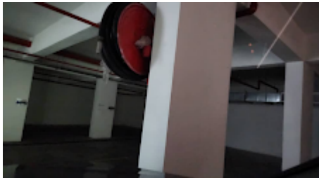
Basement Lighting 2.png
